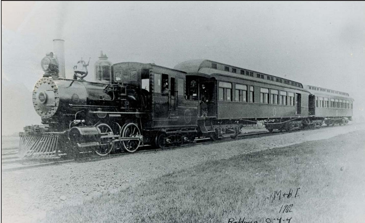
The Midlothian & Blue Island Railway was built primarily to provide transportation to a country club. The entire railroad consisted of little more than two miles of track connecting with the Rock Island Railroad. This diminutive 0-4-4T Baldwin locomotive and these two conventional railroad passenger cars began service on the line in 1901 and continued as the only equipment on the line for a decade.
